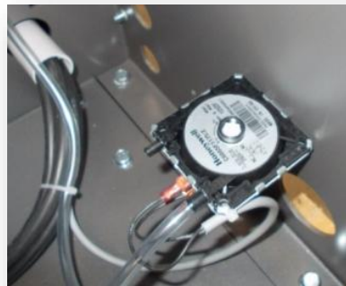
Gas pressure switch
