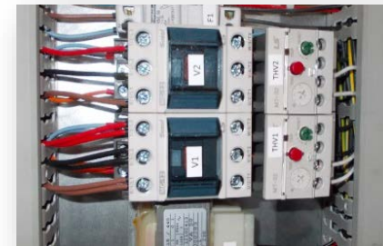
Thermic safety device
